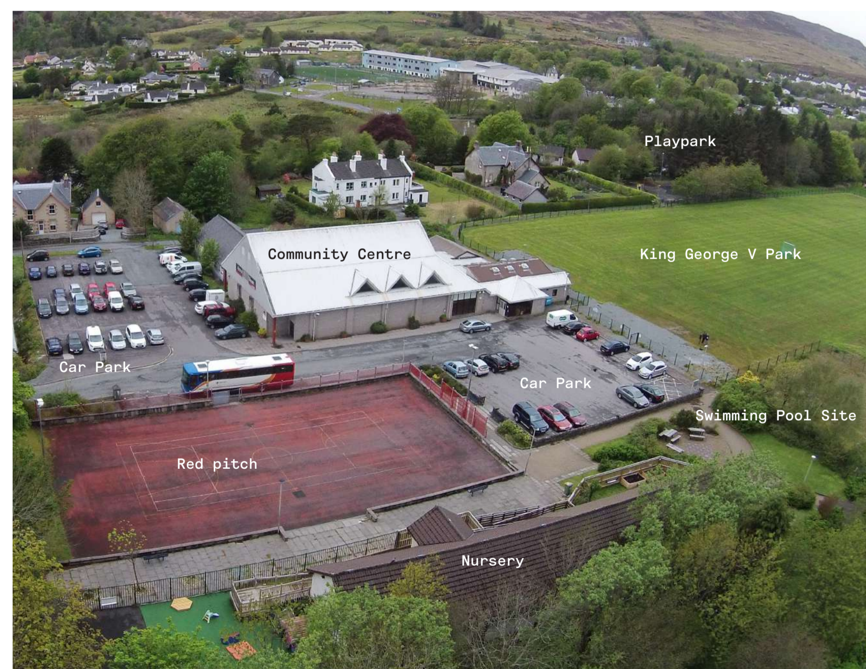
Aerial view of the site
